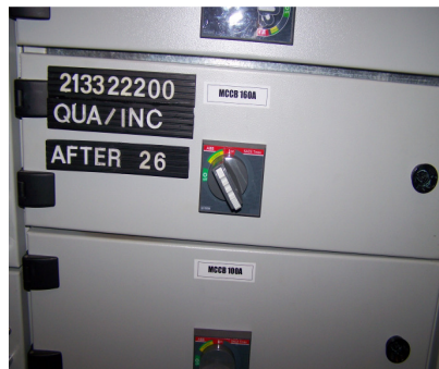
4.7b After short-circuit, the protective breaker must trip, its metal door cover must remain closed and IP be maintained
