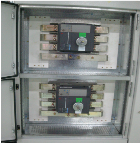
3.2.2a Each functional device i.e. breaker in Series Forti LV System is compartmentalized i.e. Form 3 and
