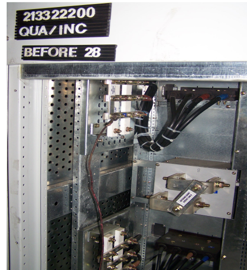
3.1.1.8 Cables and cabling accessories must be arranged to withstand short-circuit stresses and conditions
