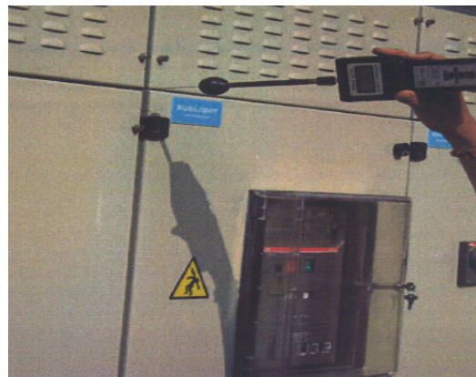
4.2d IP 4X in progress
