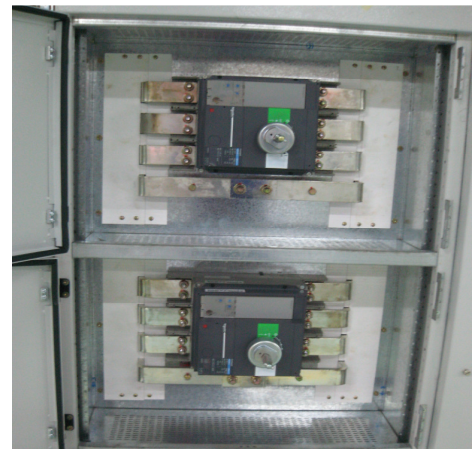
3.1.1.7a Breakers to be installed as per manufacturer's instructions, giving attention to short-circuit conditions
