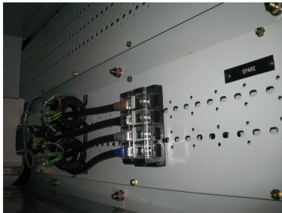
3.1.1.9a Terminal blocks are provided for external cables. Cable support provisions is catered for on the partition plate to secure the external cables
