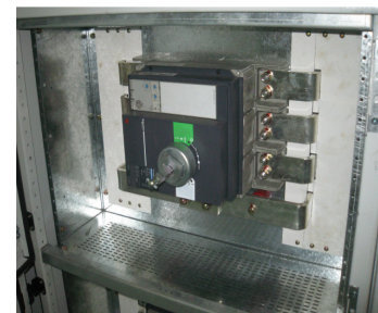
3.1.1.1 The compartment, partition and doors have to withstand the stresses during short circuit conditions
